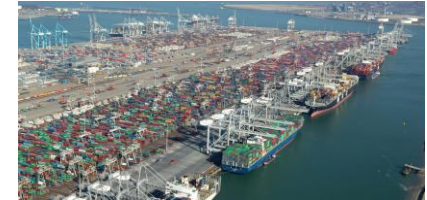
ECT (Europe Container Terminals) which is one of the most advanced container terminals in Europe.
